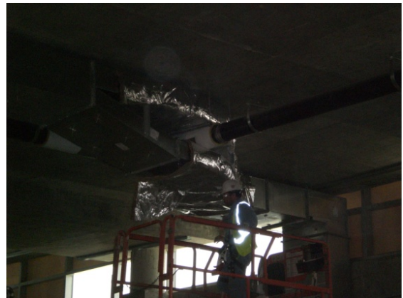
Figure 1 – 2 nd floor ductwork and plumbing clashes
